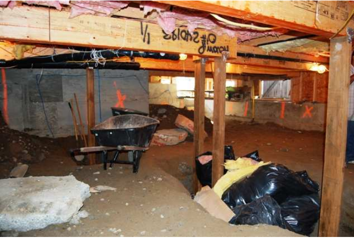
1- Excavate and install columns.
