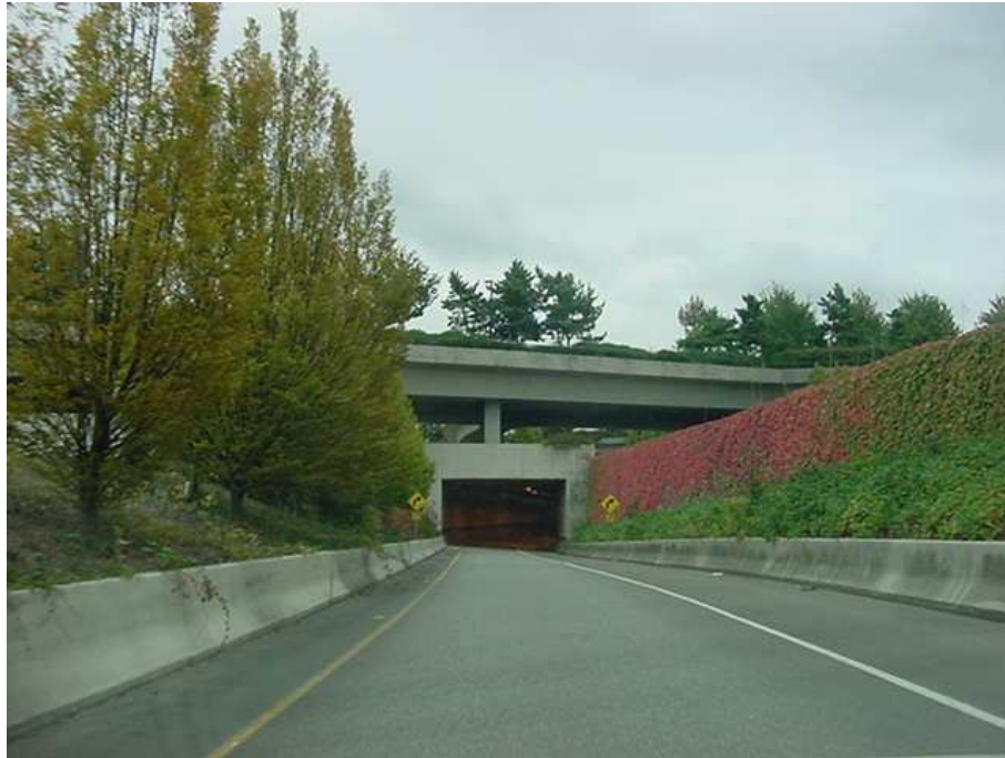
Fig 11 - Island Crest Way Tunnel Exit from I90 East from Express Freeway
