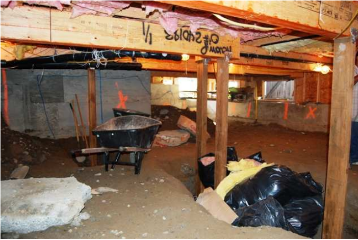
1- Excavate and install columns.
